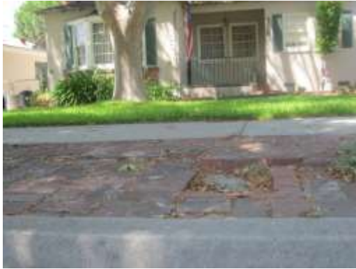
Before: Inadequately installed/maintained pavers.
