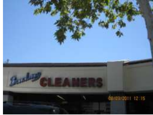
After: Façade repainted.
