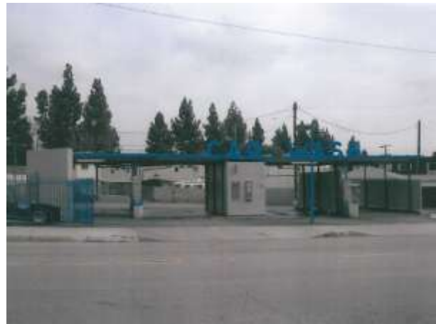
Existing car wash facility.
