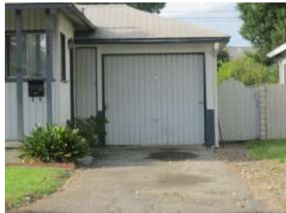
(After) Inoperable vehicle and trashcans removed.
