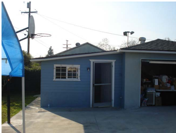
(Before) Unpermitted room addition.
