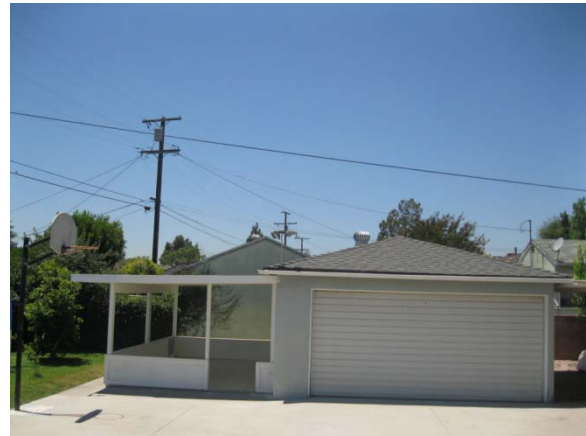
(After) Removed room addition.
