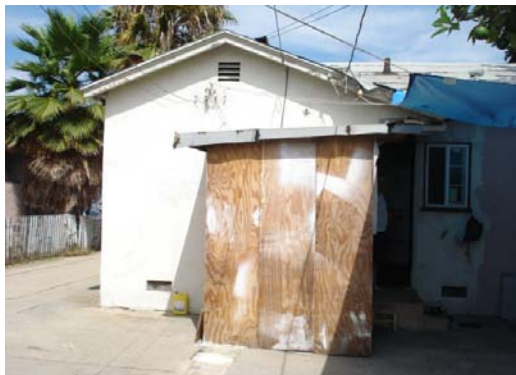
Unpermitted laundry room. (Before)
