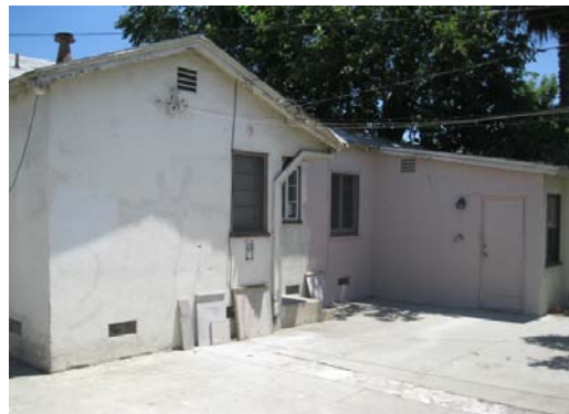
Removal of unpermitted laundry room. (After)
