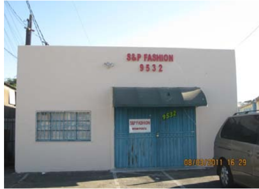
Repainted wall. (After)
