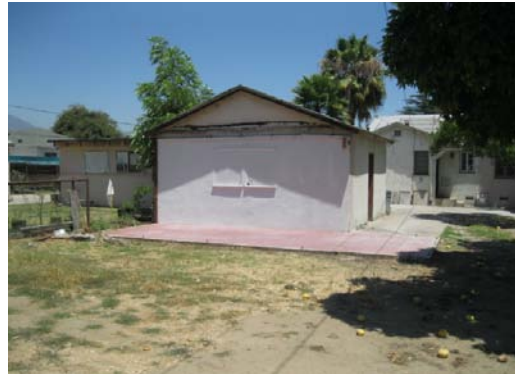
Removal of unpermitted garage room. (After)
